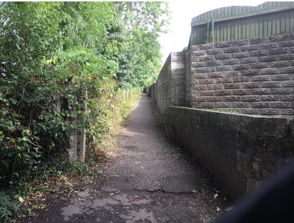
Northeastern pedestrian access point. Again, no lighting and path in very poor condition
