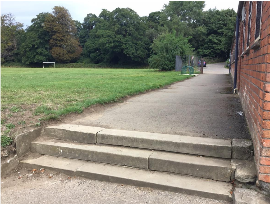
Same steps but viewed from the bottom of them
