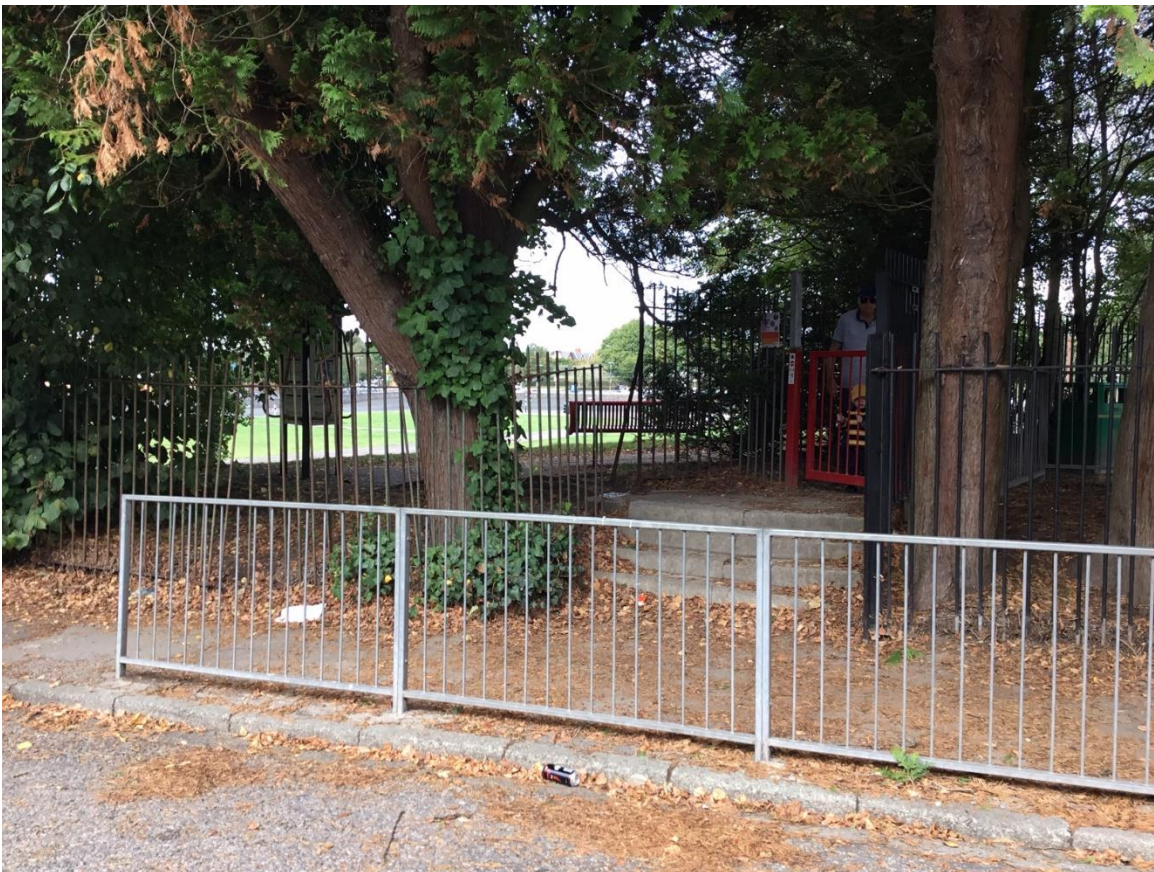
Pedestrian access from Gelligaer Street (the only access point that is not wheelchair accessible)
